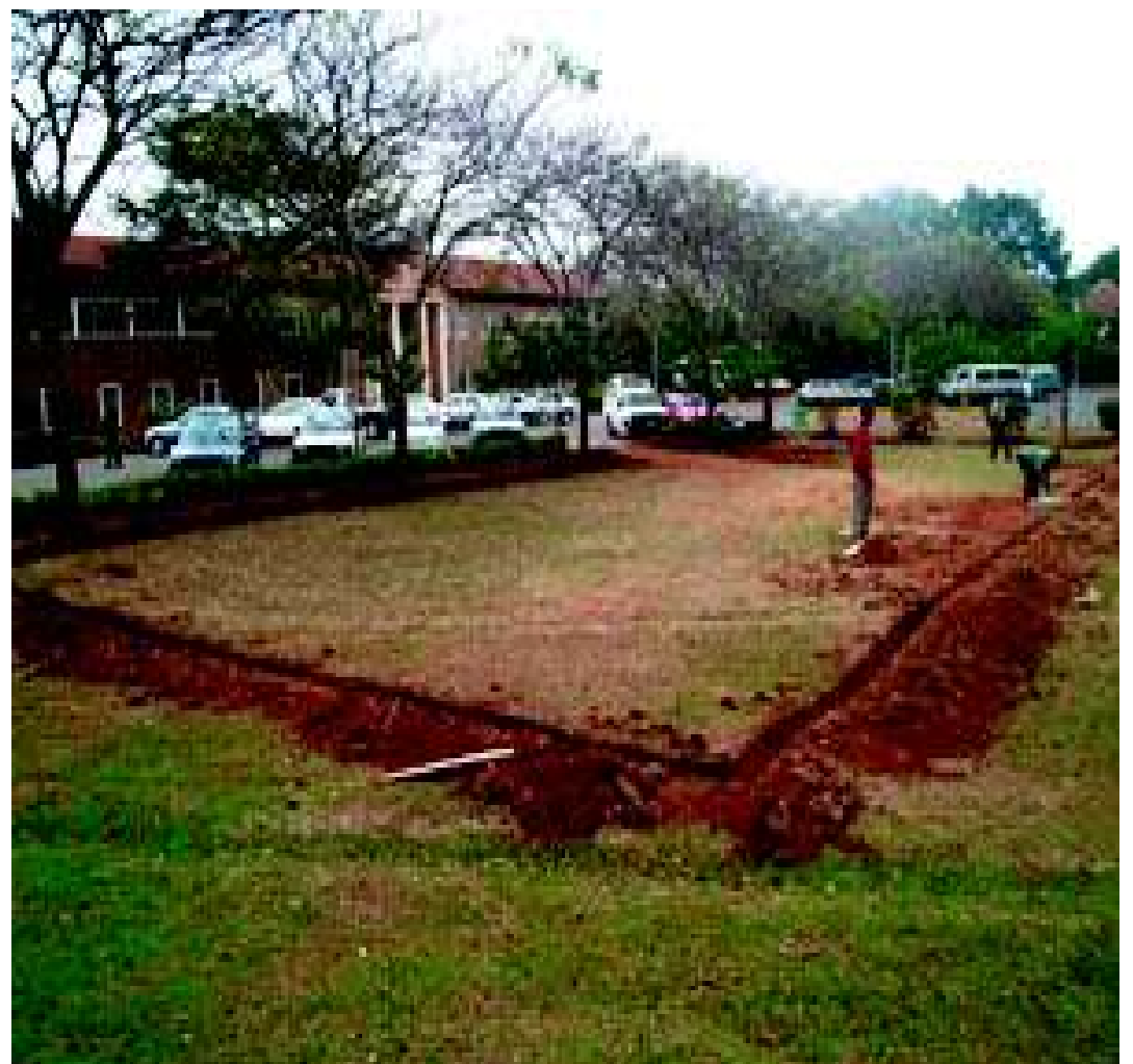
The proposed parking lot extension.
