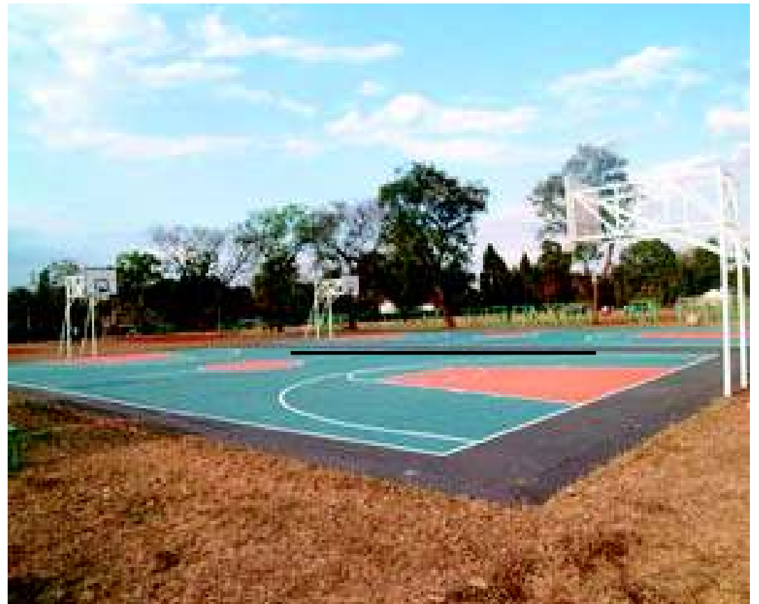
The refurbished basketball courts.
